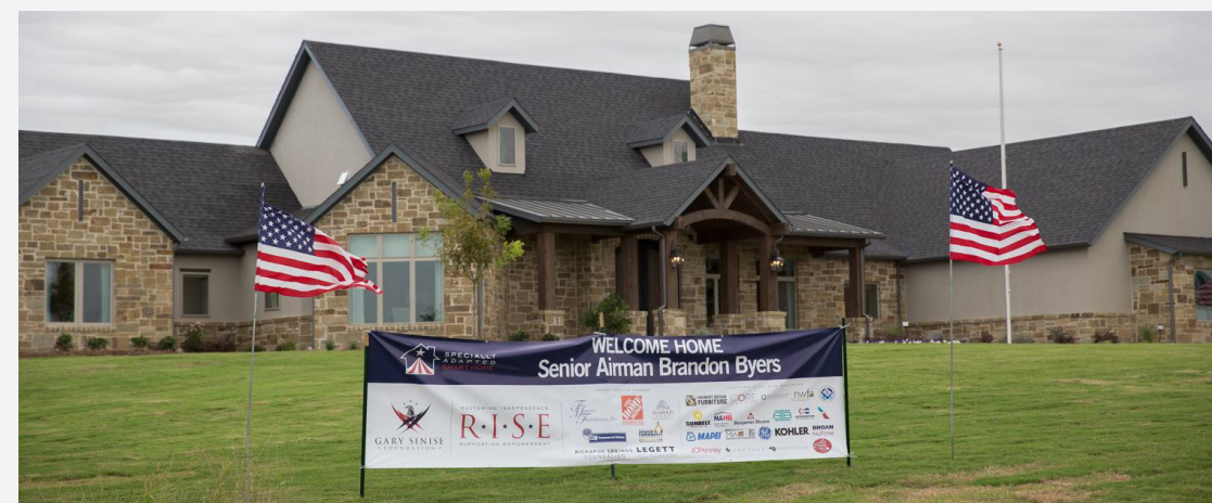
The completed Byers home awaits the dedication to the family.
